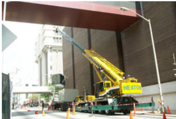
STREET CLOSURE DURING HOISTING OF AIR HANDLER UNIT
